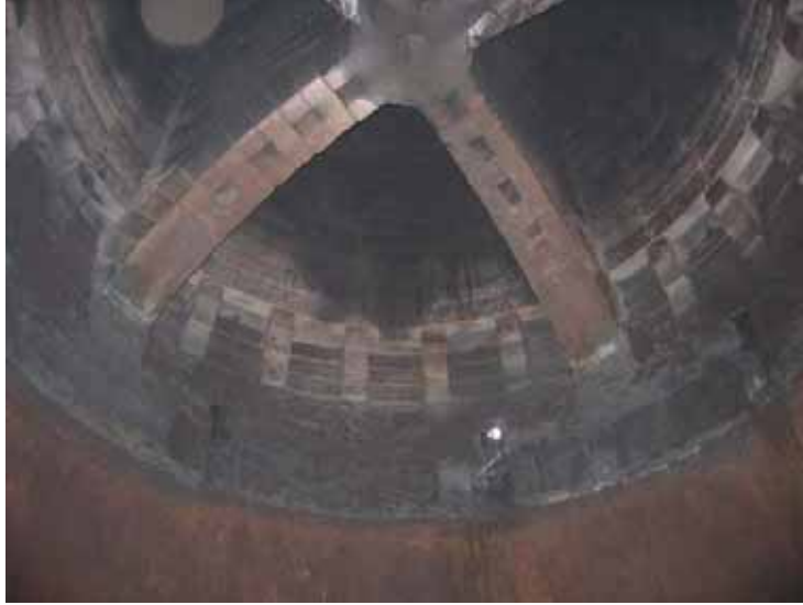
Figure 2 – Gasifier Internal Refractory
